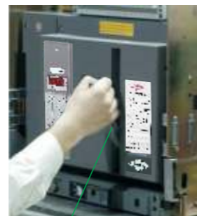
Shake with the manual energy-storage handle up and down about six times to "click".
